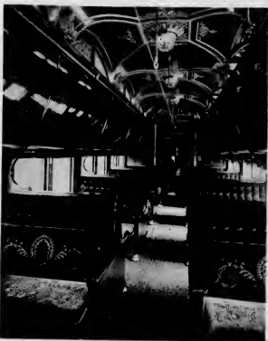
LAST CAR BUILT BY THE PULLMAN CO.
